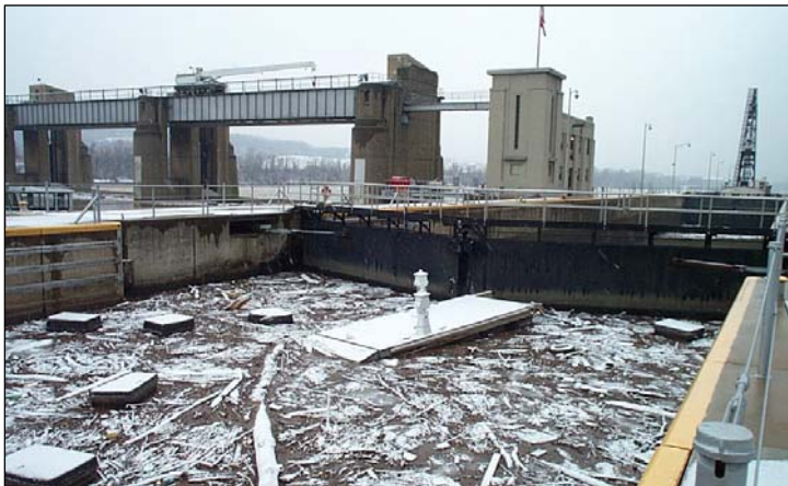
Figure 2. Debris from the McKeesport Marina trapped above Emsworth Locks and Dam on the Ohio River about six miles downstream from Pittsburgh. Photo by Andy Tuthill, ERDC-CRREL.
